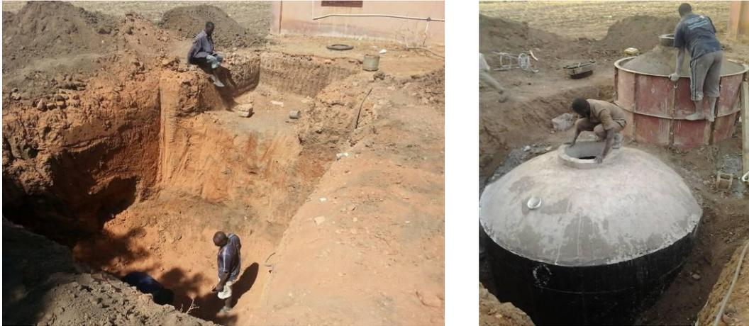
Photo – a 12 m<sup>3</sup> digester in construction in Khartoum, showing excavation and plastering of inside of main digester chamber (outflow chamber to rear)
