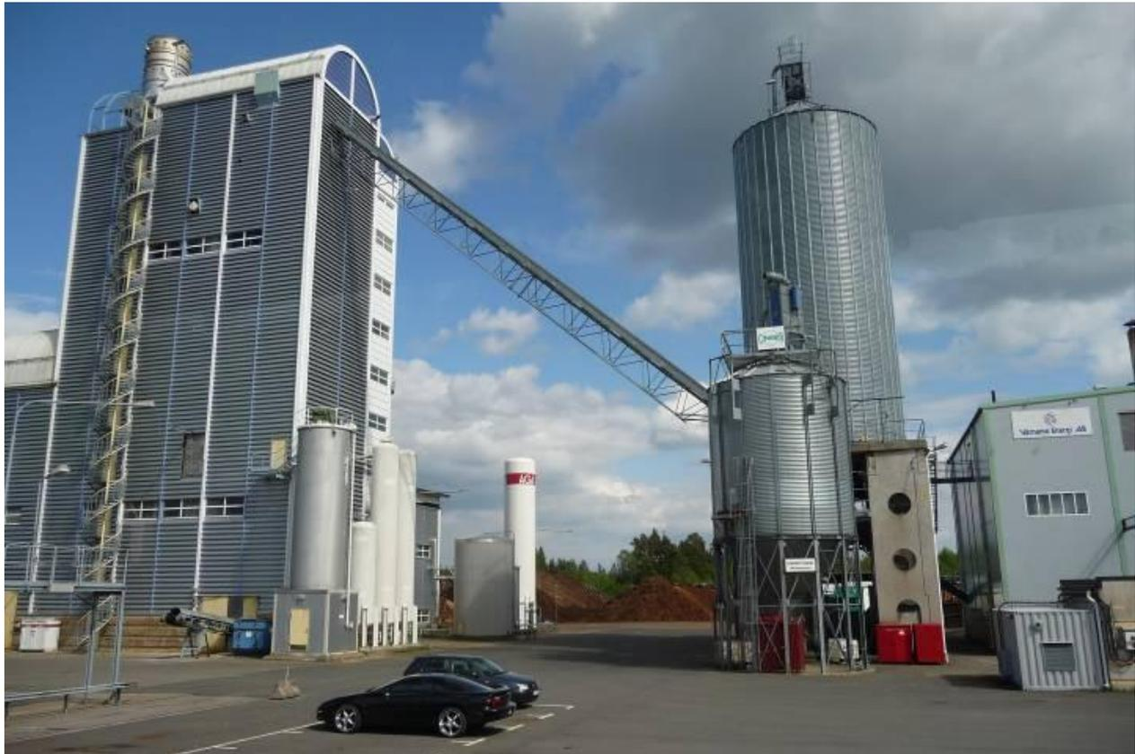
**A pilot gasification plant in Sweden – producing synthesis gas (hydrogen and carbon monoxide) from carbon rich feedstocks including wood residues and sorted municipal solid wastes**
